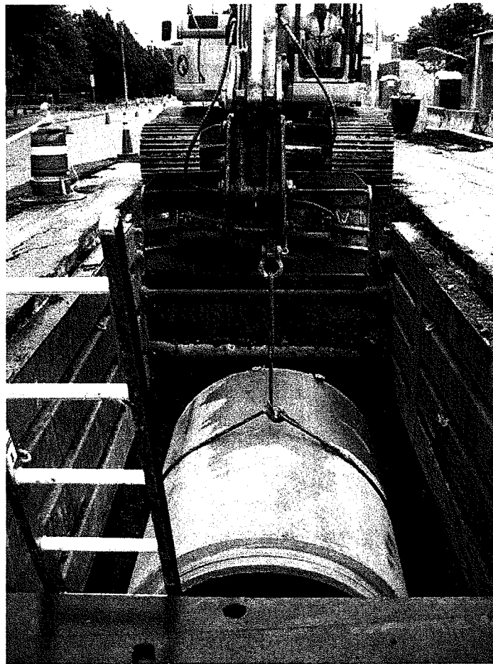
66" drain installation in Farragut Rd.
