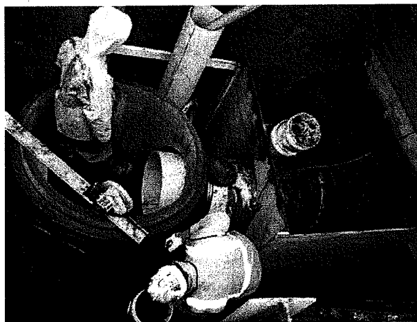
CAM400 new drain manhole at Whittemore Ave, Cambridge, MA
