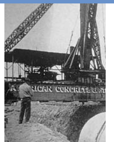
Hultman Aqueduct and Norumbega Reservoir constructed
