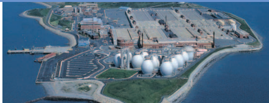
Mining of Inter-Island Tunnel between Nut Island and Deer Island completed
