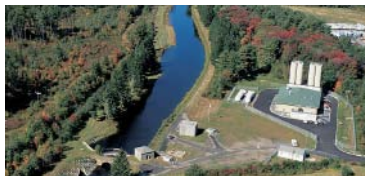
Interim Corrosion Control Facility in Marlborough completed
