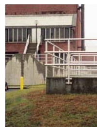
Clinton Wastewater Treatment Plant completed
