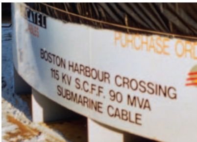
Cross-harbor power cable installed at Deer Island
