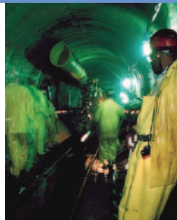
MetroWest Water Supply Tunnel groundbreaking
