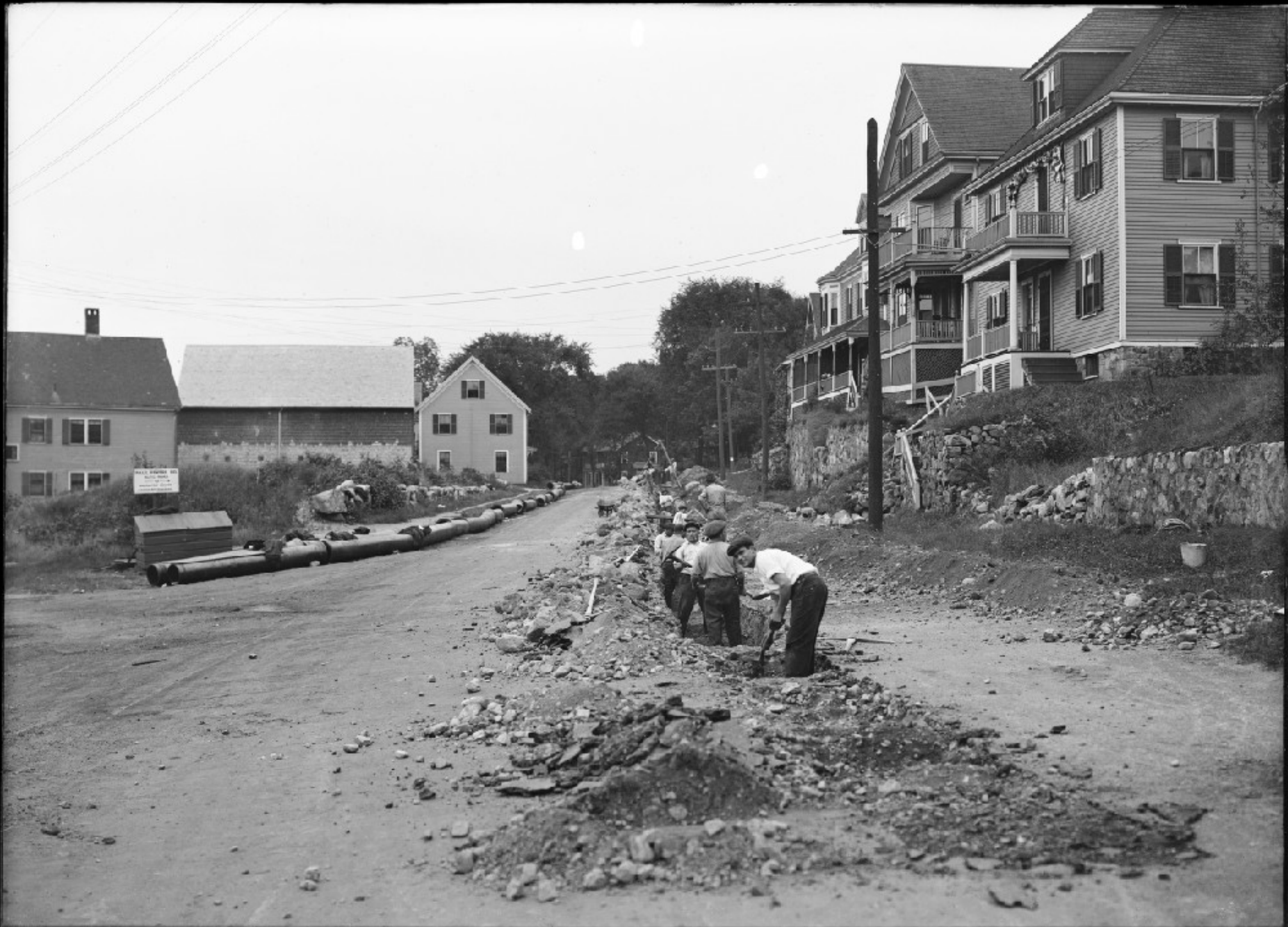
N. EX. H. 8. P. L. SEC. 45 ARLINGTON. 16 IN. PIPE TRENCH COR. OF MASS. AV. & PAUL REVERE RD. SEPT. 15, 1919. 7585
