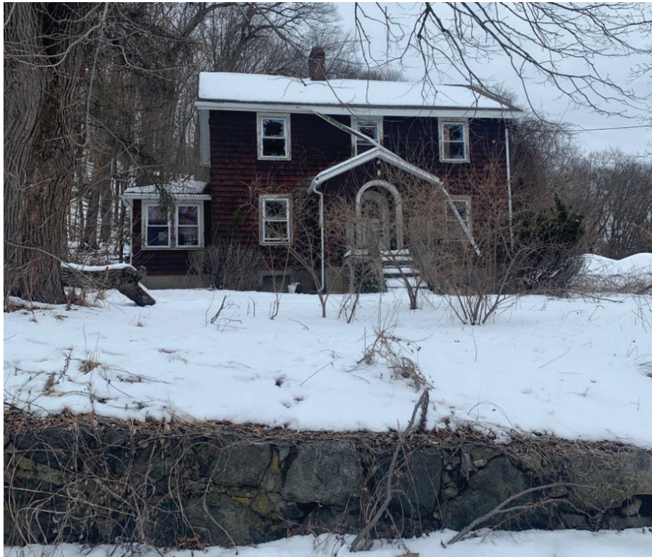
17. Lower Fernald Property Site – south-facing façade of Cottage #20 – Staff Residence (WLT.734) proposed for demolition in Alternative 10A.
