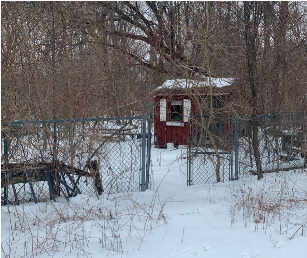
10. Lower Fernald Property Site – looking west towards shed (WLT.788)
