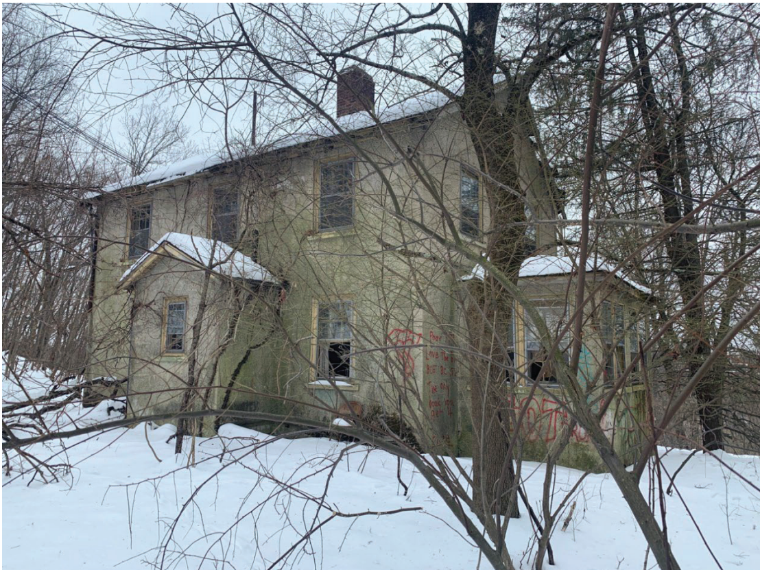
15. Lower Fernald Property Site – rear (north) and west elevations of Cottage #18 – Staff Residence (WLT.732)
