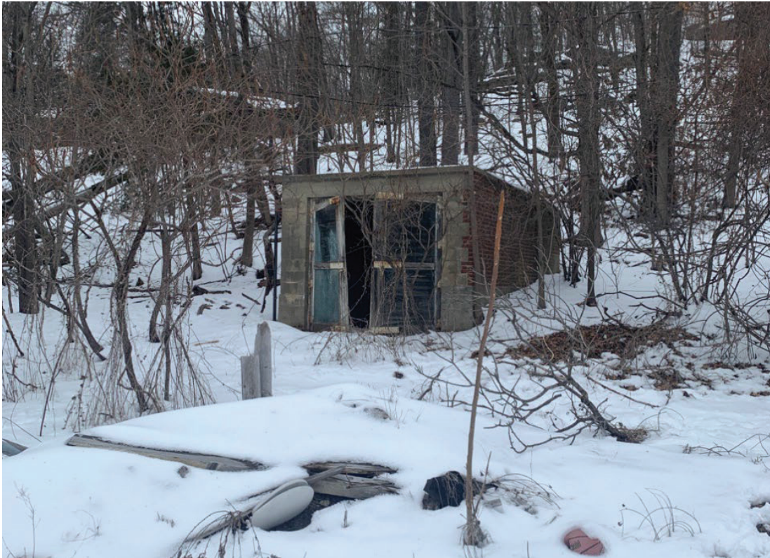
18. Lower Fernald Property Site – south-facing façade and east elevation of garage (WLT.769)
