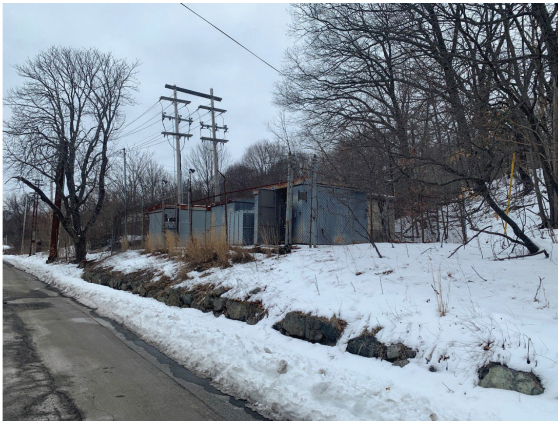
11. Lower Fernald Property Site – view northwest toward electric substation (WLT.740)
