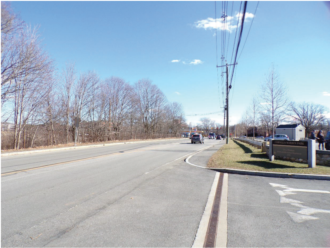
1. UMass Property Site – view east towards Waverley Oaks Road showing UMass Property Site (left) and Cornelia Warren Park (right)
