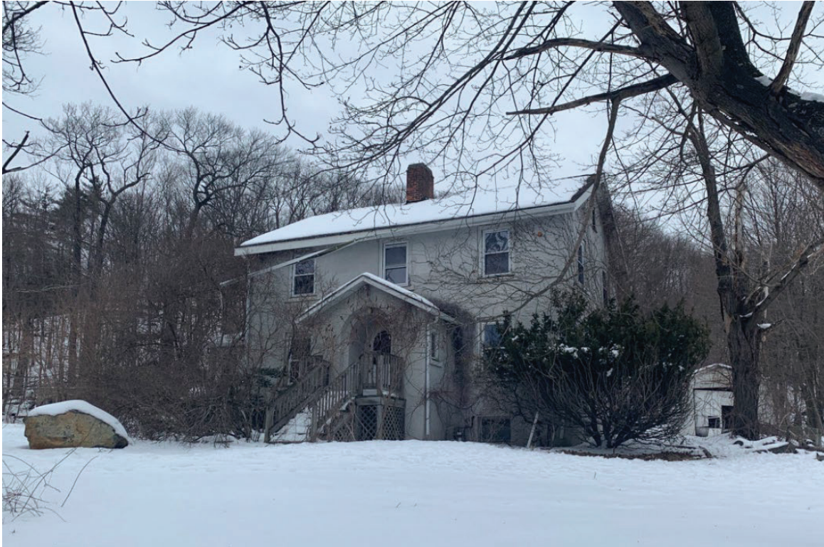
16. Lower Fernald Property Site – View east showing Cottage #19 – Staff Residence (WLT.733; foreground) and Garage (WLT.770; background) proposed for demolition in Alternative 10A.
