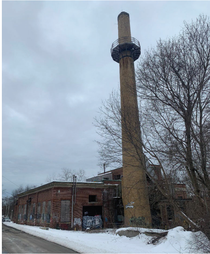
12. Lower Fernald Property Site – north and west elevations of power plant (WLT.935)
