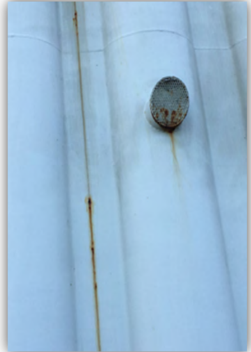
Vertical seams and vent
