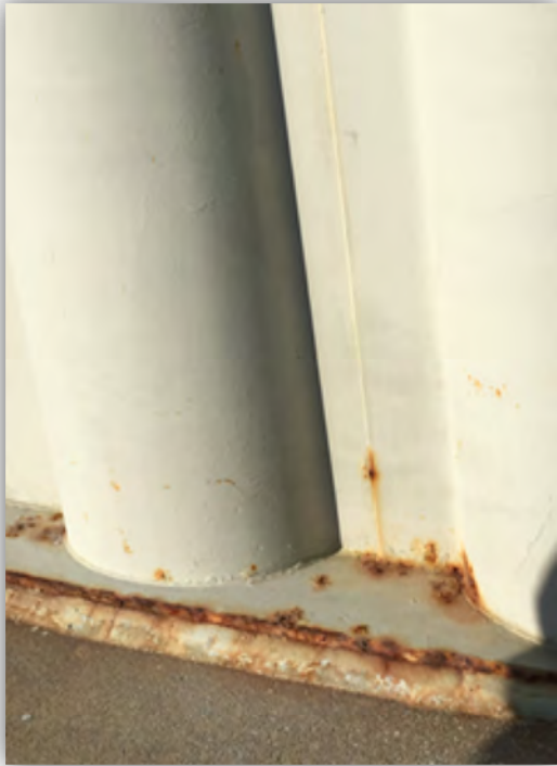
Bottom of tank fluted column at foundation
