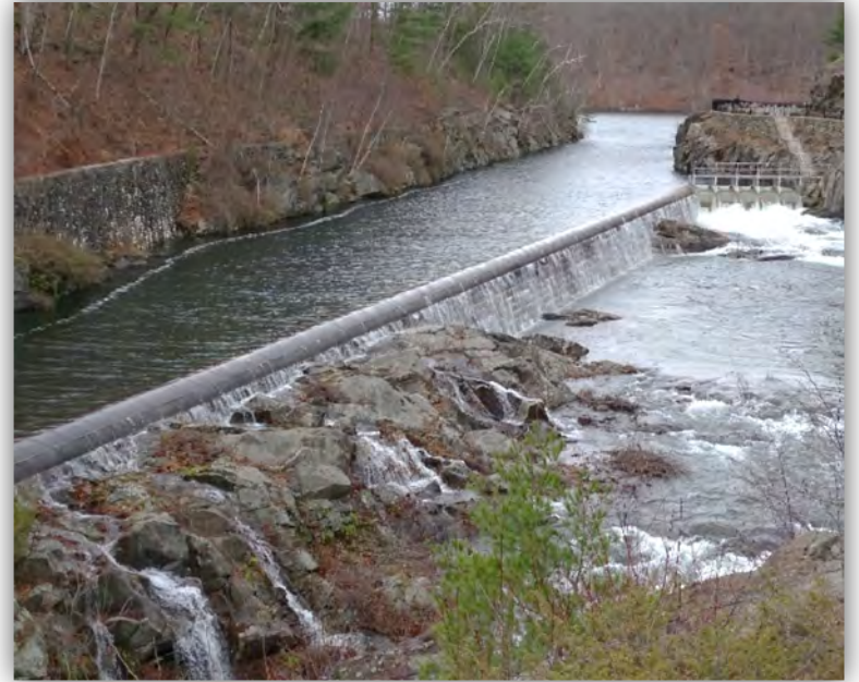
Quabbin Spillway, December 31, 2018
