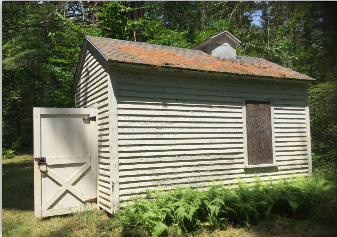
Well Pump House
