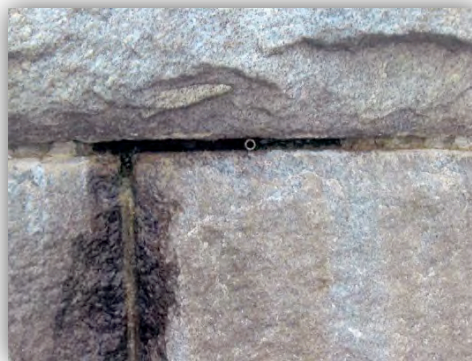
Missing mortar
