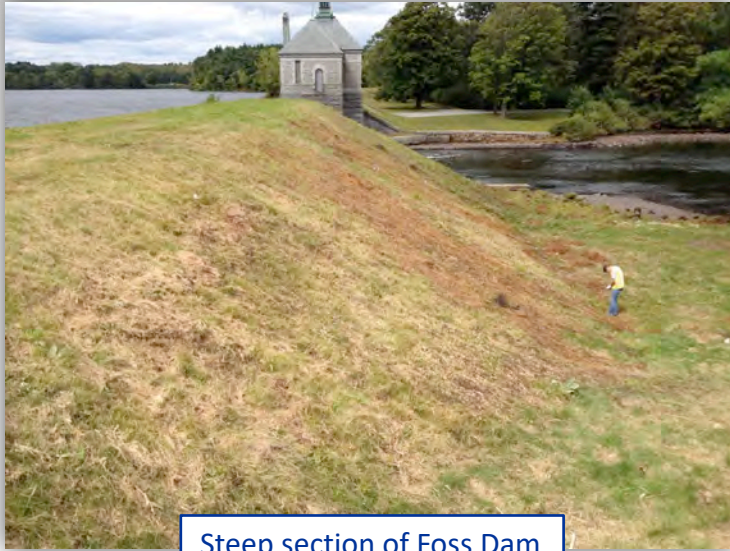
Example of armoring turf protection
