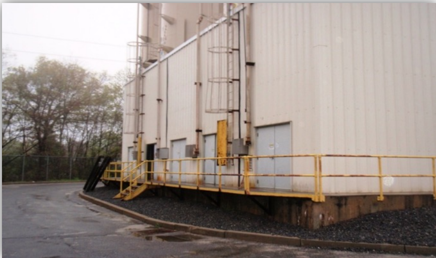
Soda Ash Storage
