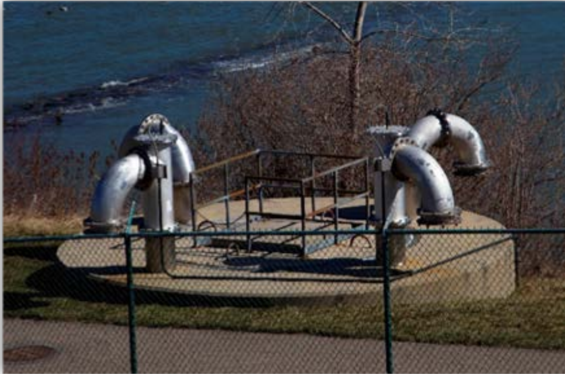
South System Shaft at Nut Island Headworks
