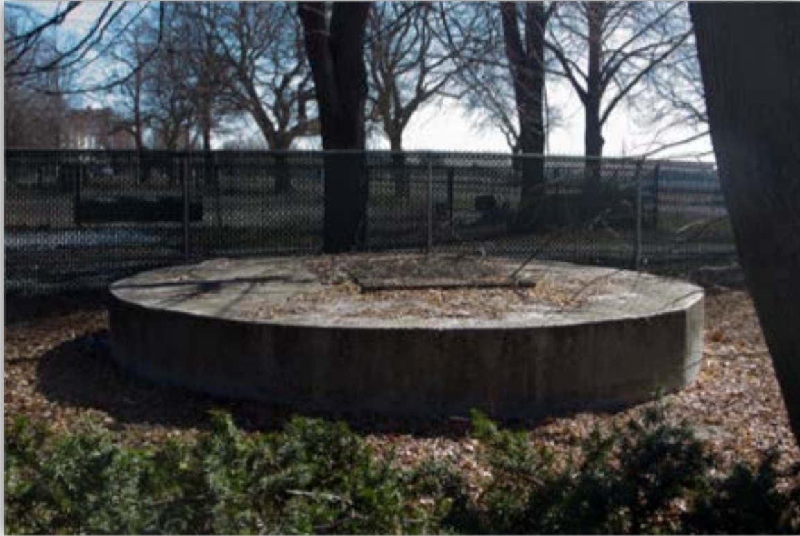
Top of Effluent Shaft at Columbus Park Headworks
