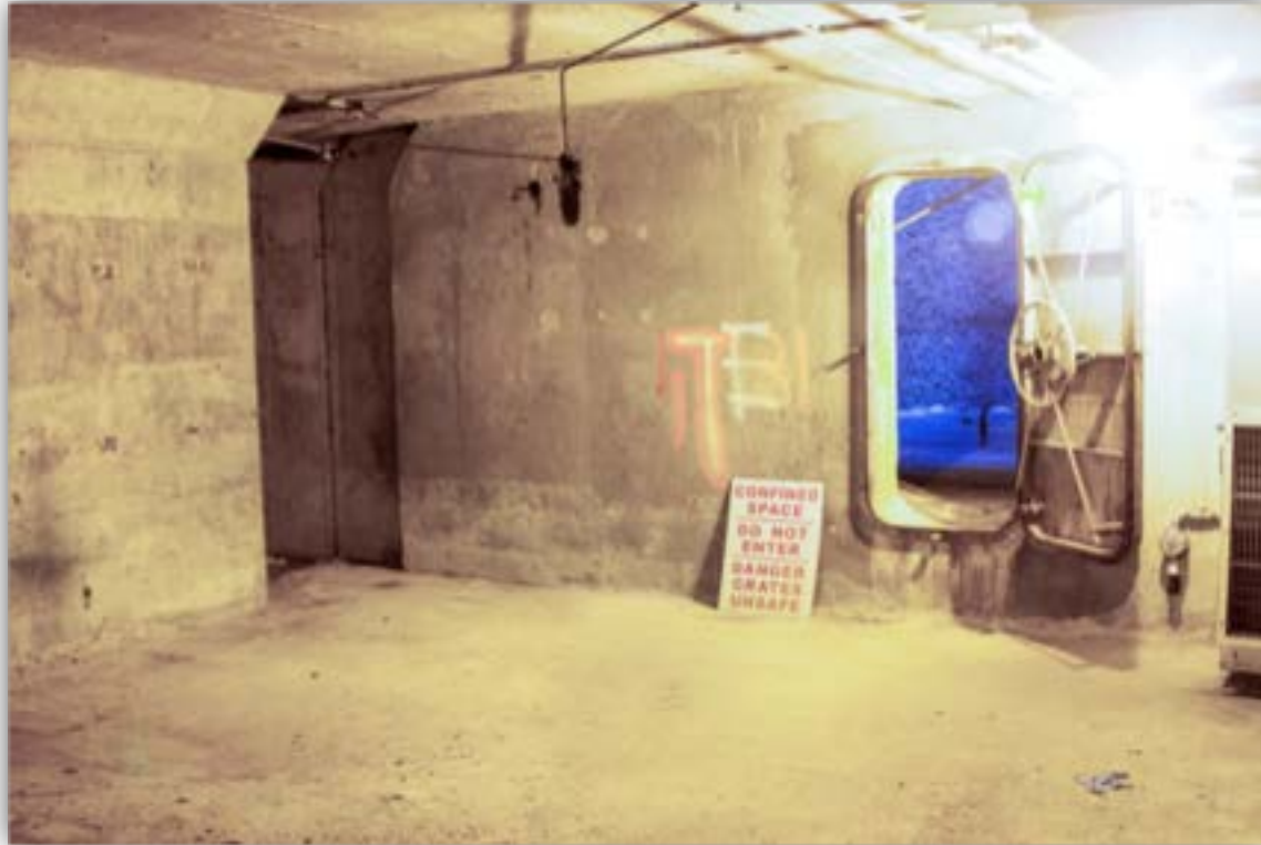
Doorway from Connecting Structure into Shaft at Chelsea Creek Headworks
