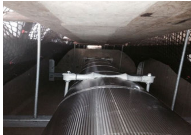
Stainless Steel Pipe Below Rt. 9 Bridge.
