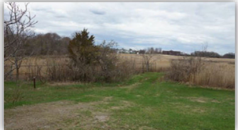
Shaft 7D located near salt marsh at Neponset River Reservation
