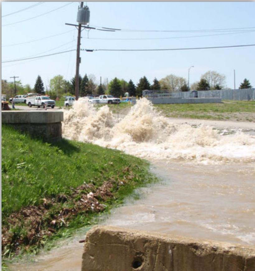
250 MGD flow at Shaft 5 break....
