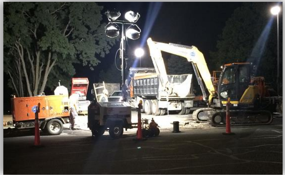
Night work on 36-inch NIH pipeline in Woburn (2016)
