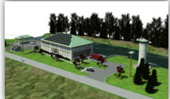
Wachusett Aqueduct Pump Station
