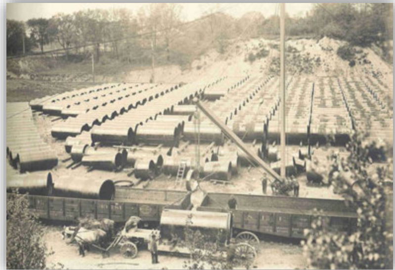
WASM 1 and 2 Pipe Yard (1915)
