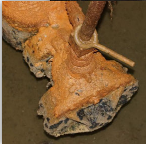
Gear box on valve at Shaft 8
