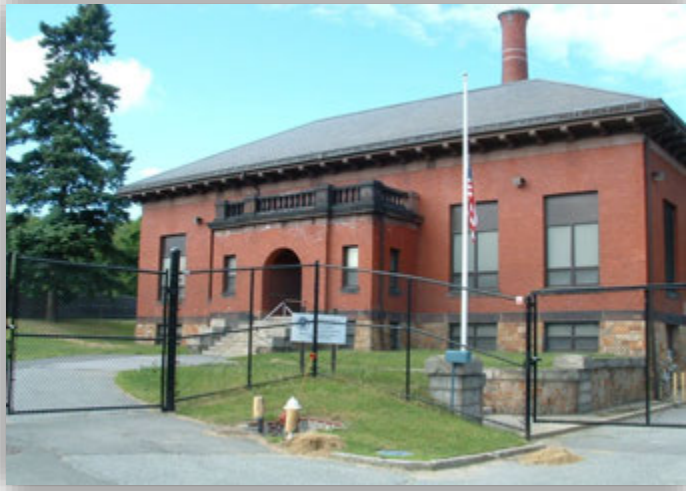
Brattle Court Pump Station (1907)
