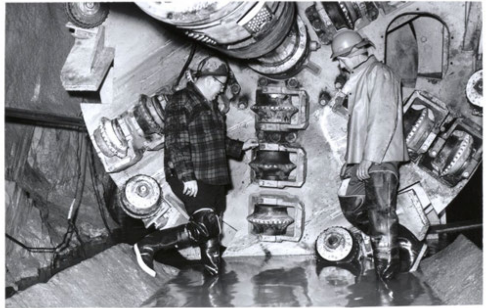
Mole cutter bits Dorchester Tunnel
