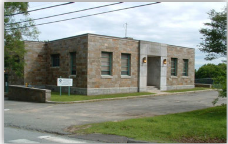
Spring Street Pump Station (1958) redundancy to Brattle Court
