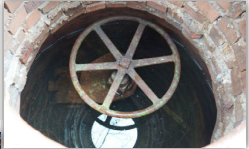
Shaft 7C connection to Section 58
