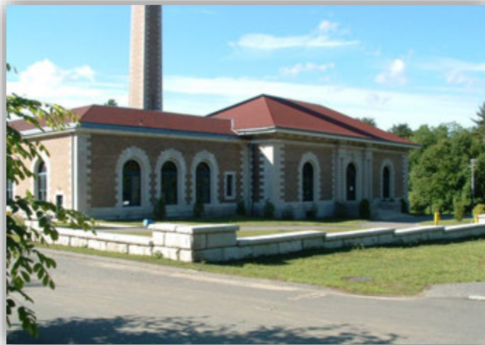
Gillis Pump Station (1899)
