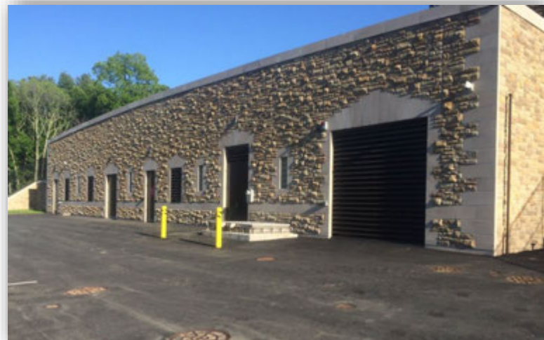
Spot Pond Pump Station (2015) redundancy to Gillis Station
