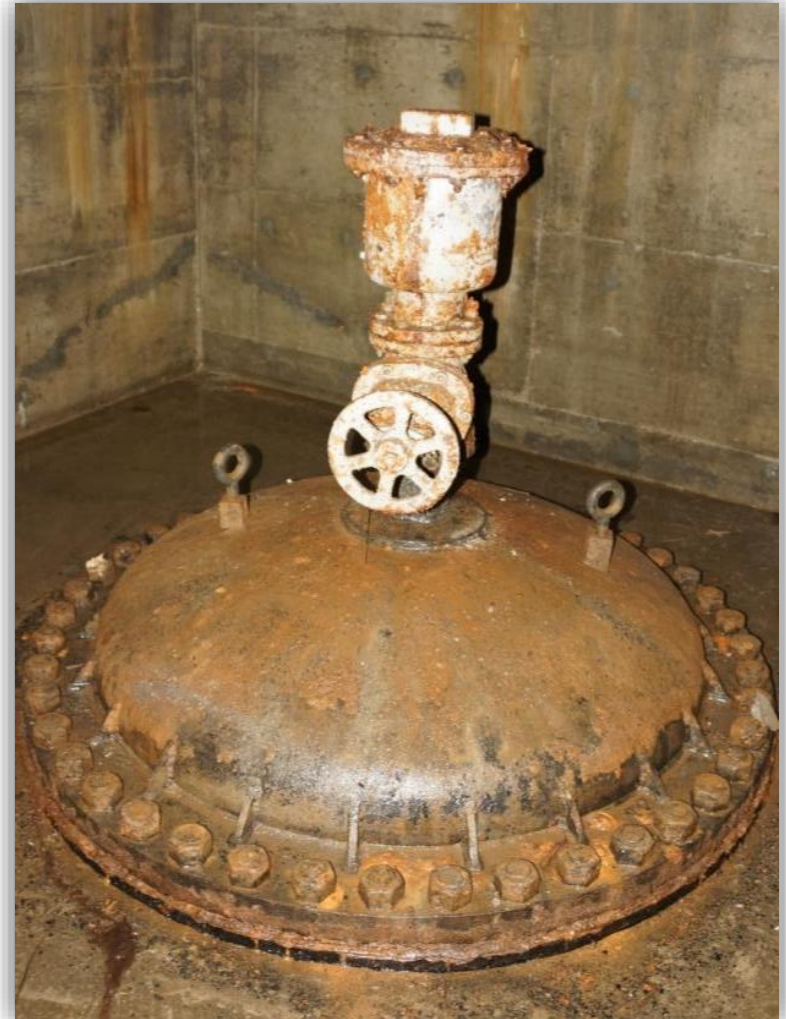
Top of Shaft 8
