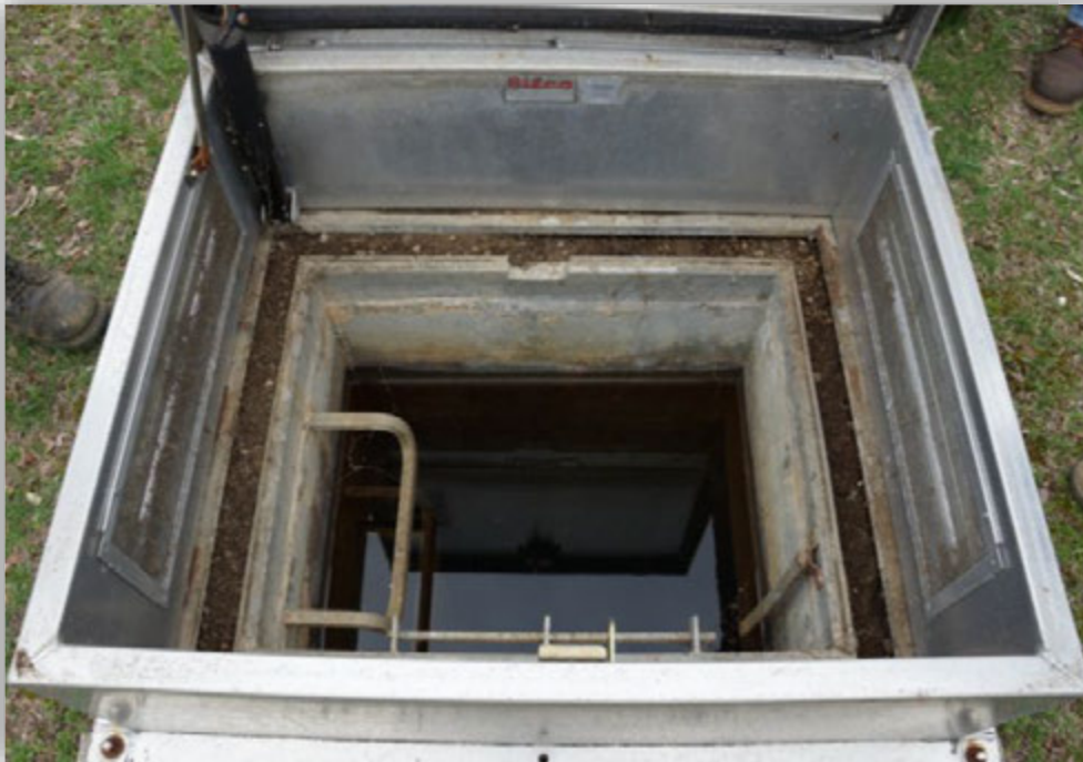
Chamber at Shaft 7C
