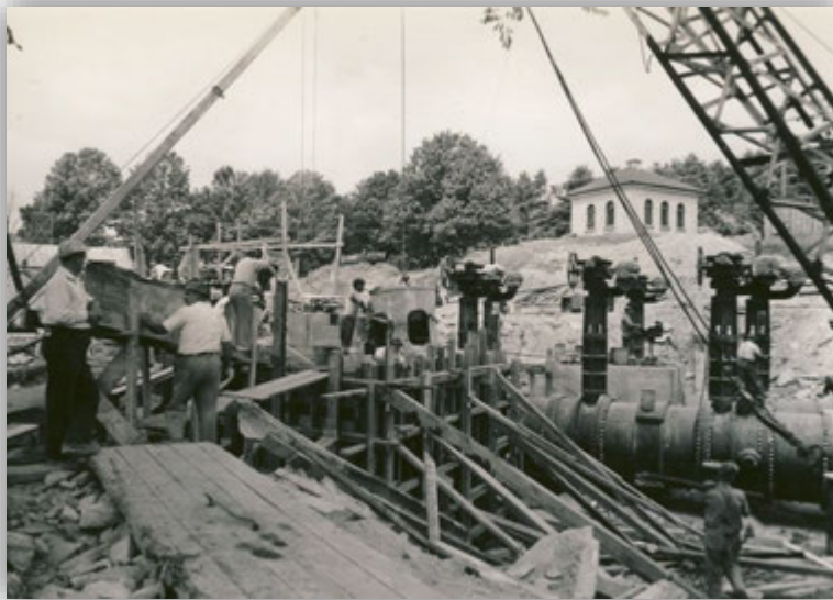
Future Hultman Aqueduct connection at Shaft 4 (1940)
