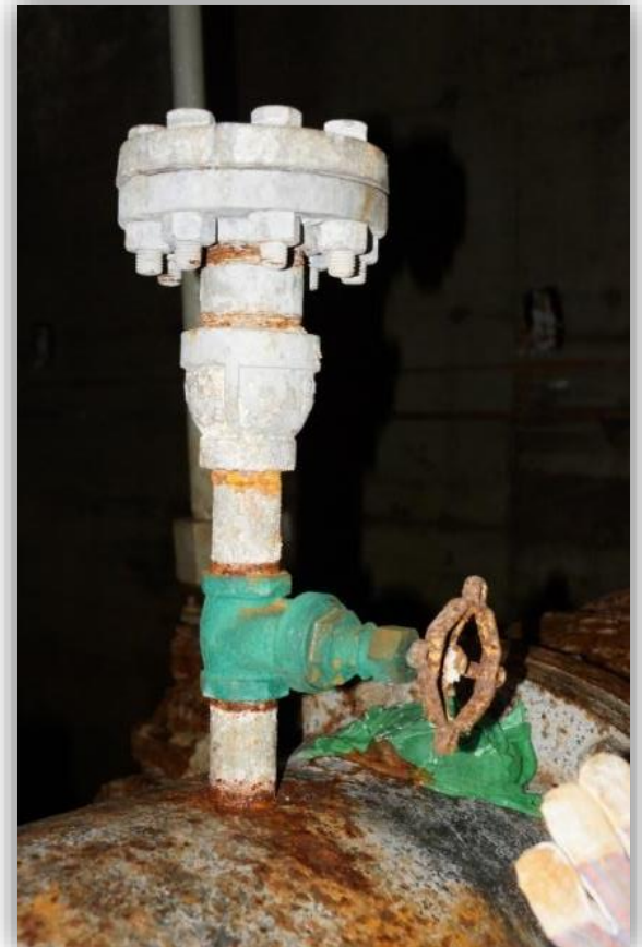
Shaft 8 PRV Chamber
