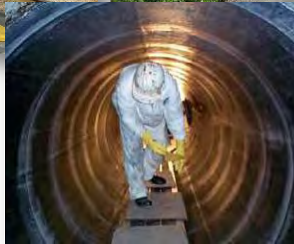
CFRP Installation
