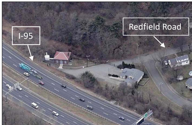
Figure 1: Hayes Pump Station
