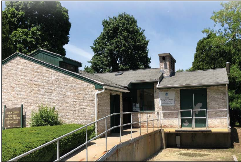
Figure 2: Hayes Pump Station
