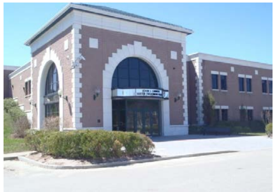
John J Carroll Water Treatment Plant
