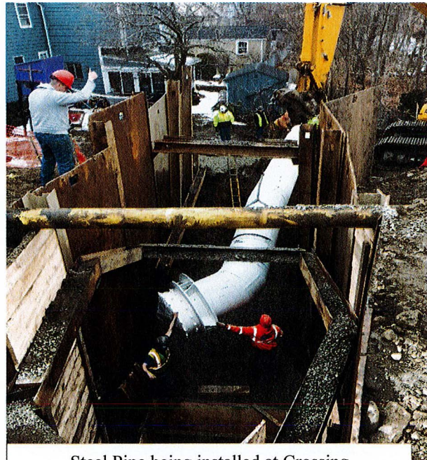
Steel Pipe being installed at Crossing
