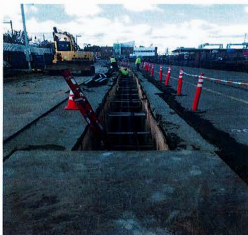
Figure 2 - Excavation Conley Terminal
