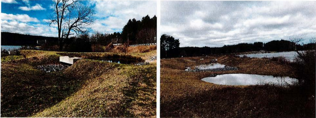
Wachusett Reservoir Direct Discharge Elimination System basins
