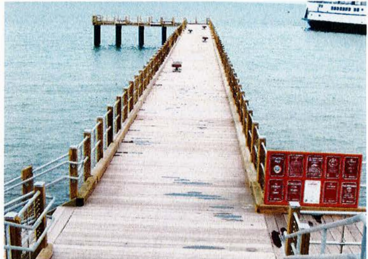
Similar Pier Installed in Oak Bluffs
