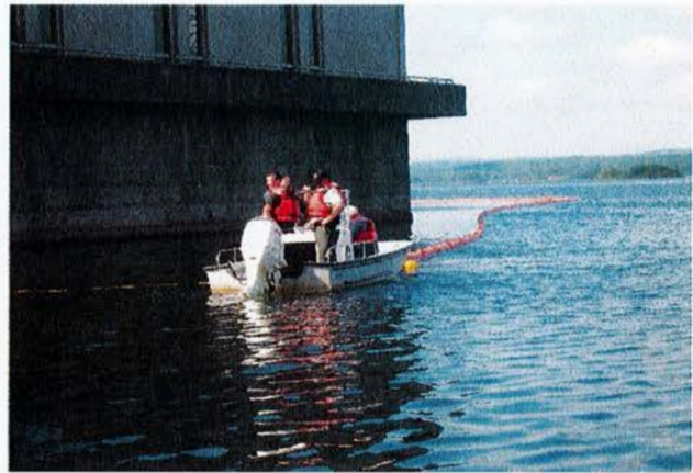
Shoreline anchor (L) and Boom enclosing Cosgrove Intake (R)
