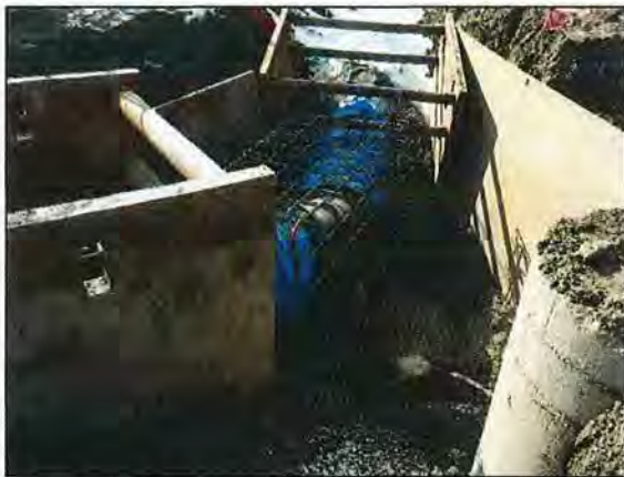
Additional reinforcing steel installed at thrust block.
