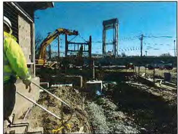
Stone bedding and filter fabric along length of pipe.
