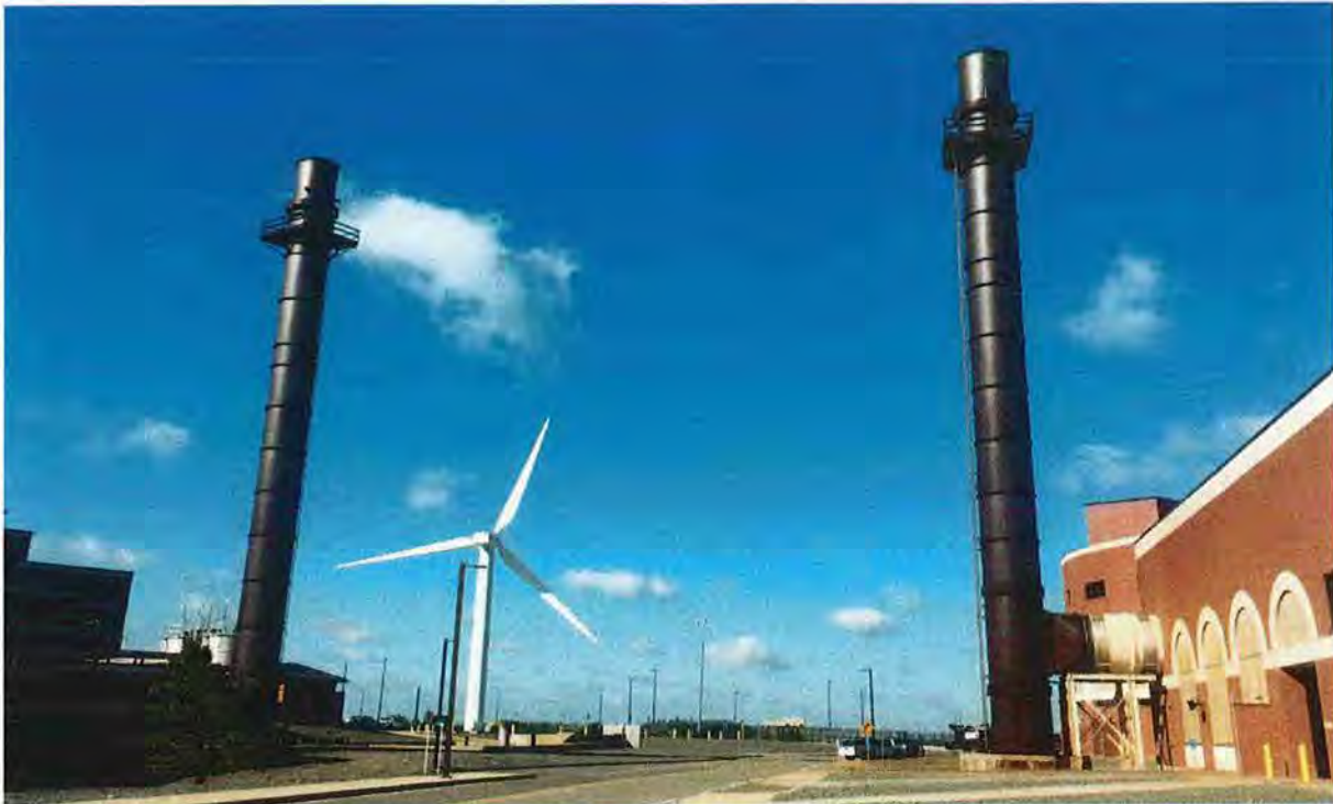
Deer Island Odor Control Emission Stacks
