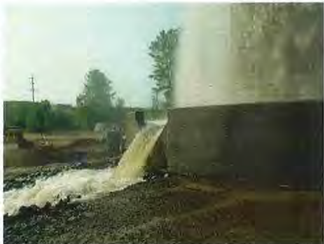
Surge Tank Overflow
