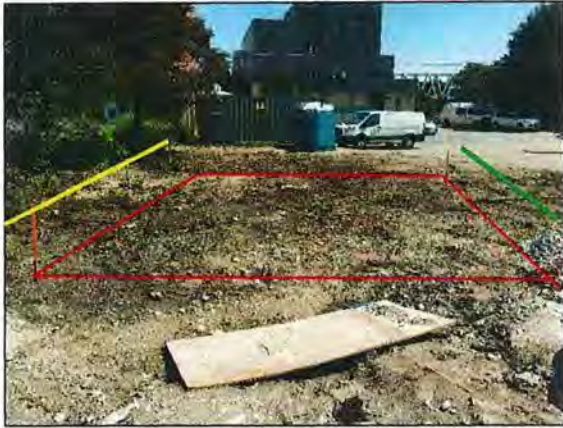
Proposed microwave antenna tower footprint (red) and 24-inch gas main (yellow) and MWRA sewer (green)
