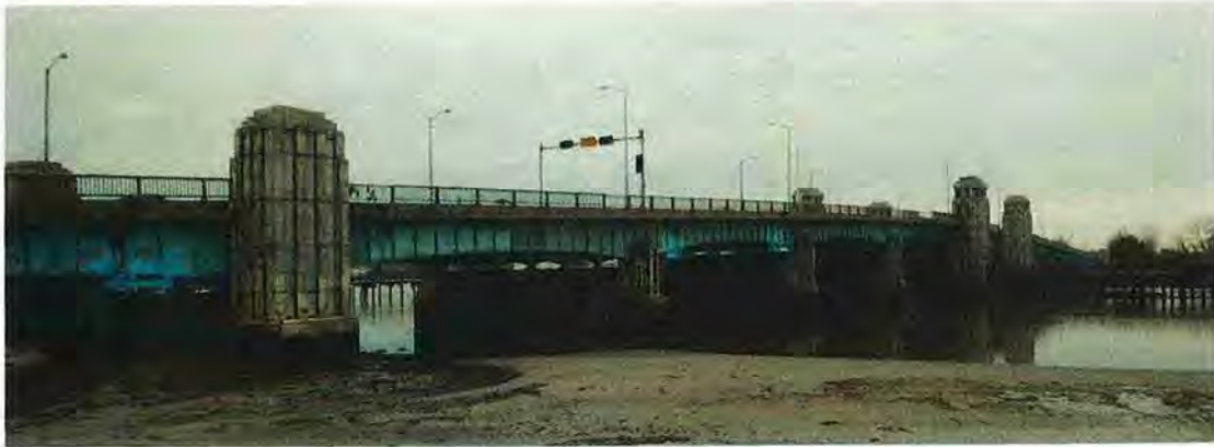
Figure 1 – General Edwards Bridge, East Elevation.
