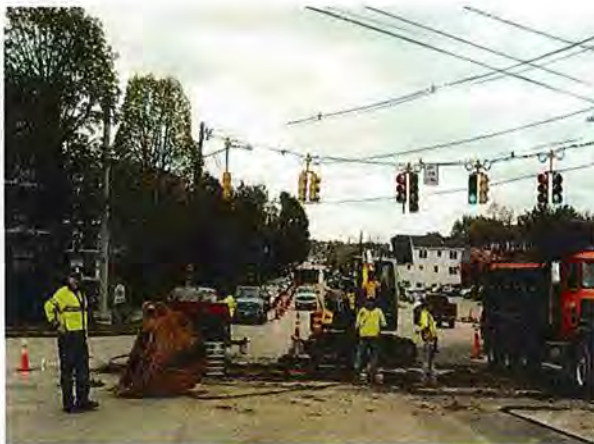
Police Details at intersection of Main Street and North Street
