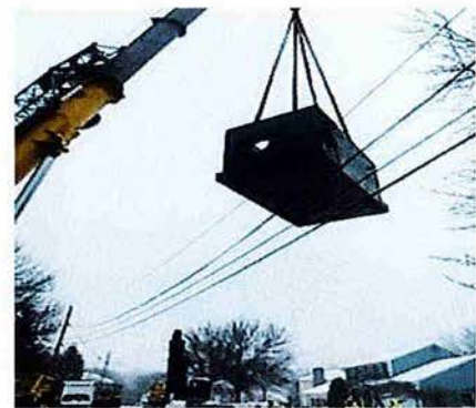
Crane lowering valve vault into place at Leach park
