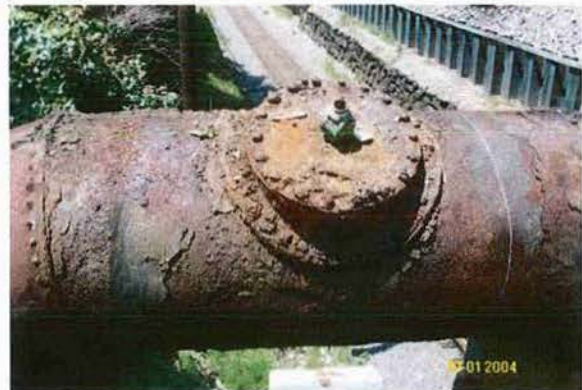
Waltham Bridge Pipeline before replacement
