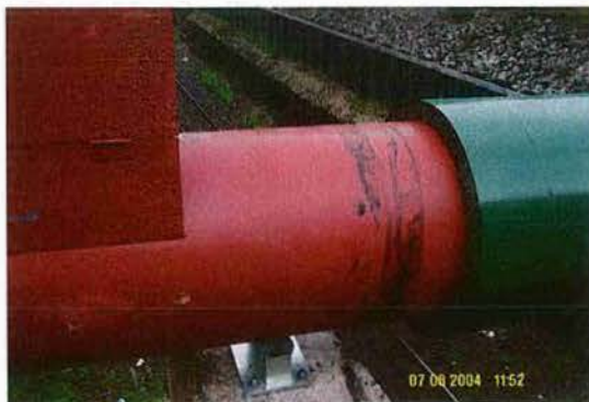
Waltham Bridge Pipeline Replaced 2004
