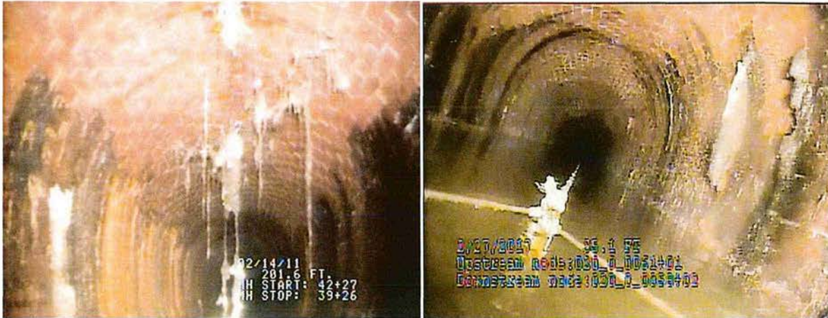
Figures 4 and 5. Sections 20/21 existing conditions.
