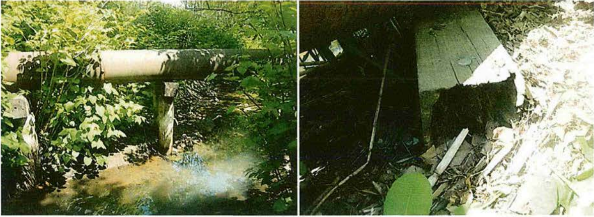
Figures 2 and 3. Water Section 50 on Wood supports at Winter Brook, Medford.
