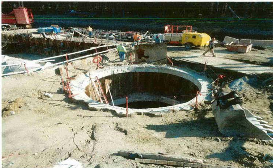
Surge Tank Excavation
