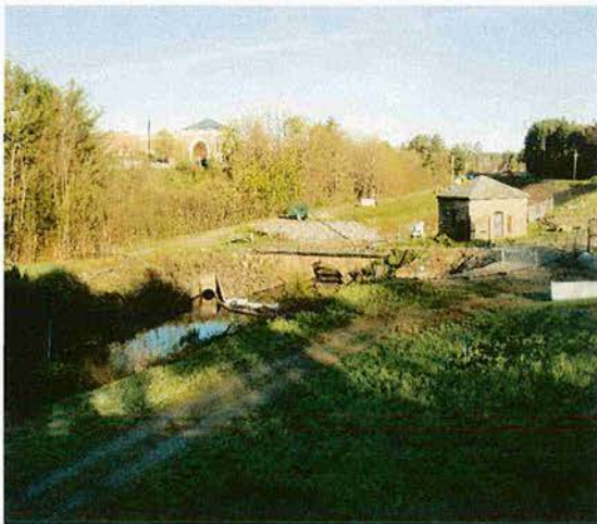
Hultman Intake Building
