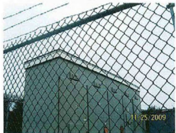
Membrane Roof on Outdoor Switchgear.
