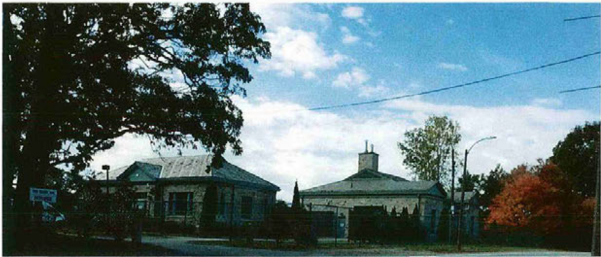
Commonwealth Avenue Pump Station, Newton
