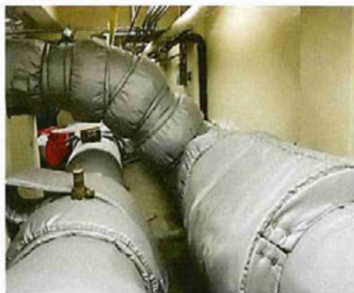
Insulation of Water Piping
