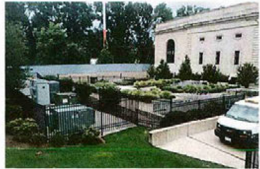
Figure 4: The top of the Emergency Pump Station with the low service condominiums in the background
