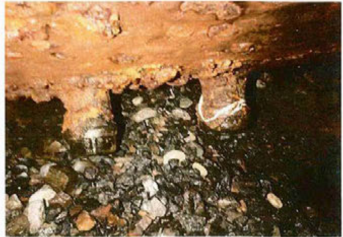
Cap Welded Over Plug
