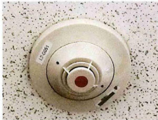
Replace Smoke Detector
