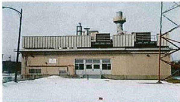
Existing east side of facility
