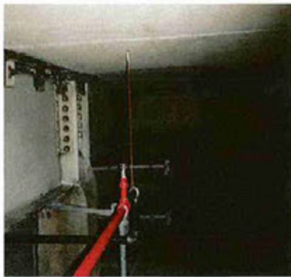
Sprinkler Head and Piping Replacement
