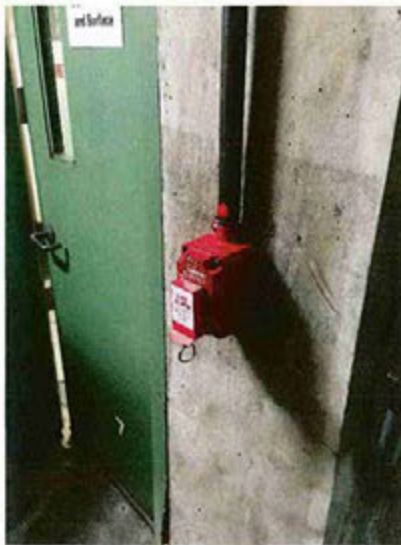
Replace Fire Alarm Pull Station
