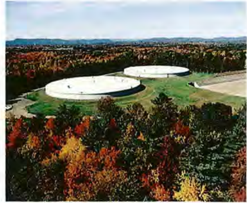
Nash Hill Water Storage Tanks
