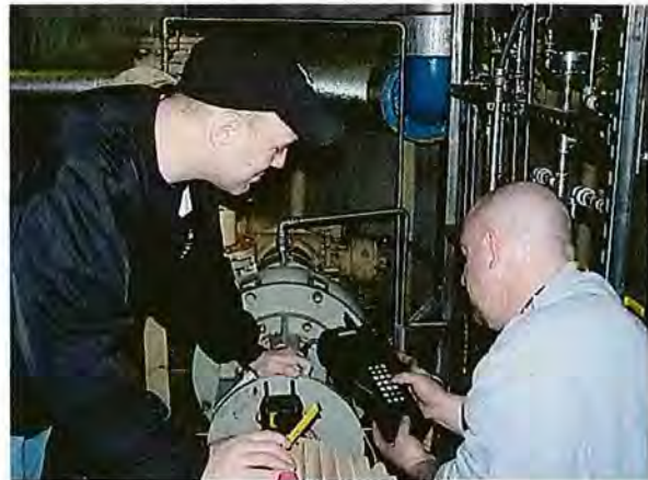
Aligning a Pump
