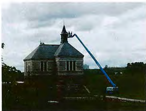
Repairing Cupola Roof on the Foss Reservoir Gatehouse
