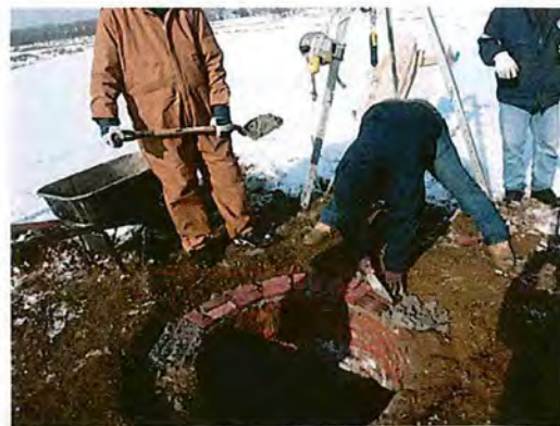
Masonry Work on a Manhole
