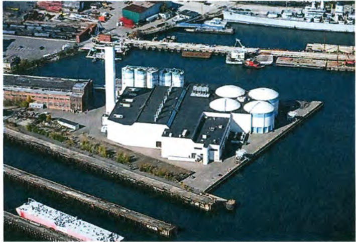
Figure 1: MWRA's Biosolids Processing Plant
