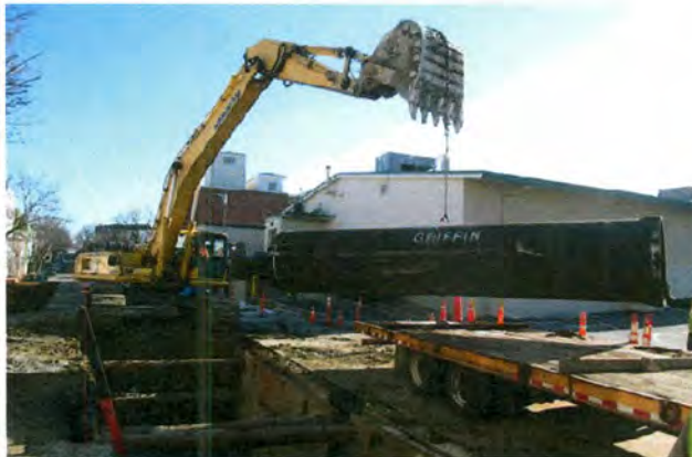
Installation of 48" drain on East Third Street Reserved Channel Contract 3B
