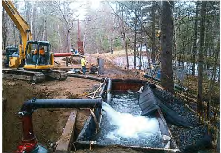
Figure 3. 12-Inch Outlet into Detention Basin
