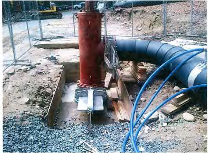
Figure 1. 36-Inch Line stop with Bypass
