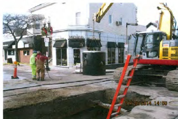
Drain manhole installation, K Street at East Broadway Reserved Channel Contract 4
