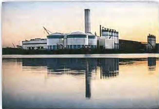
Figure 1: MWRA's Pelletizing Plant
