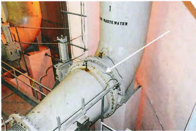
Lower 60-inch Butterfly Valve in NMPS
