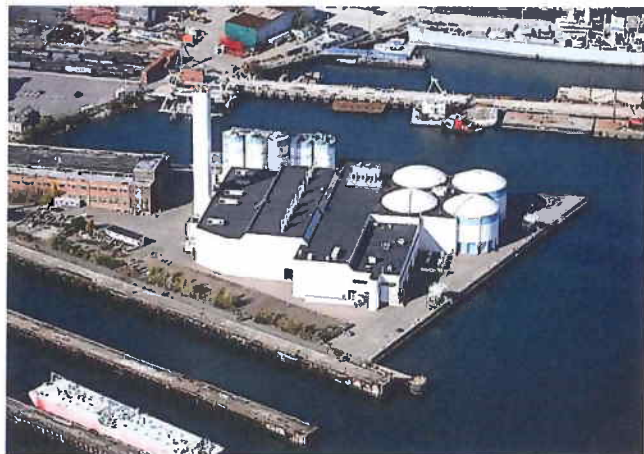
Figure 3: MWRA Pelletizing Plant at FRSA
