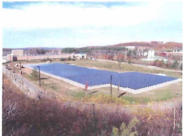
476 kW photovoltaic system at Carroll
