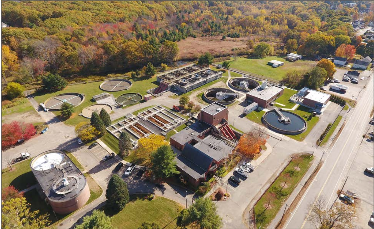
Clinton Wastewater Treatment Plant
