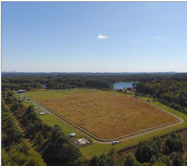
Norumbega Covered Storage Facility in Weston
