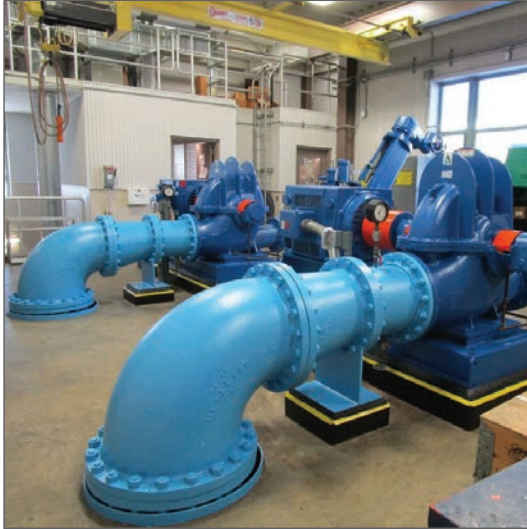
Commonwealth Avenue Pumping Station, Newton
