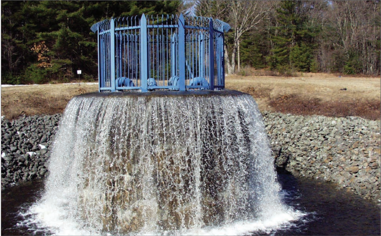
Quabbin Shaft 2 Overflowing
