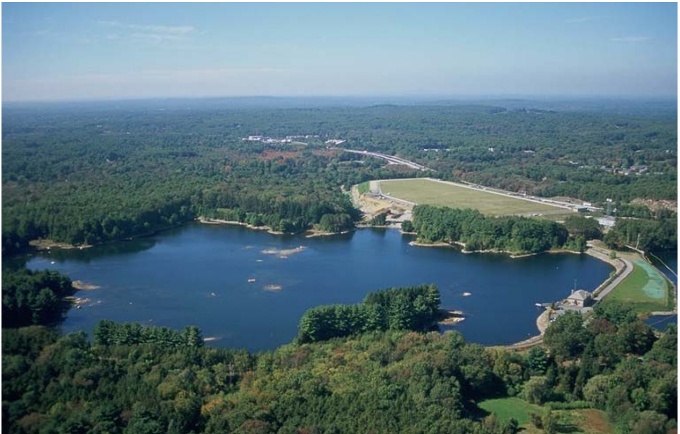
Norumbega Covered Storage Tank
