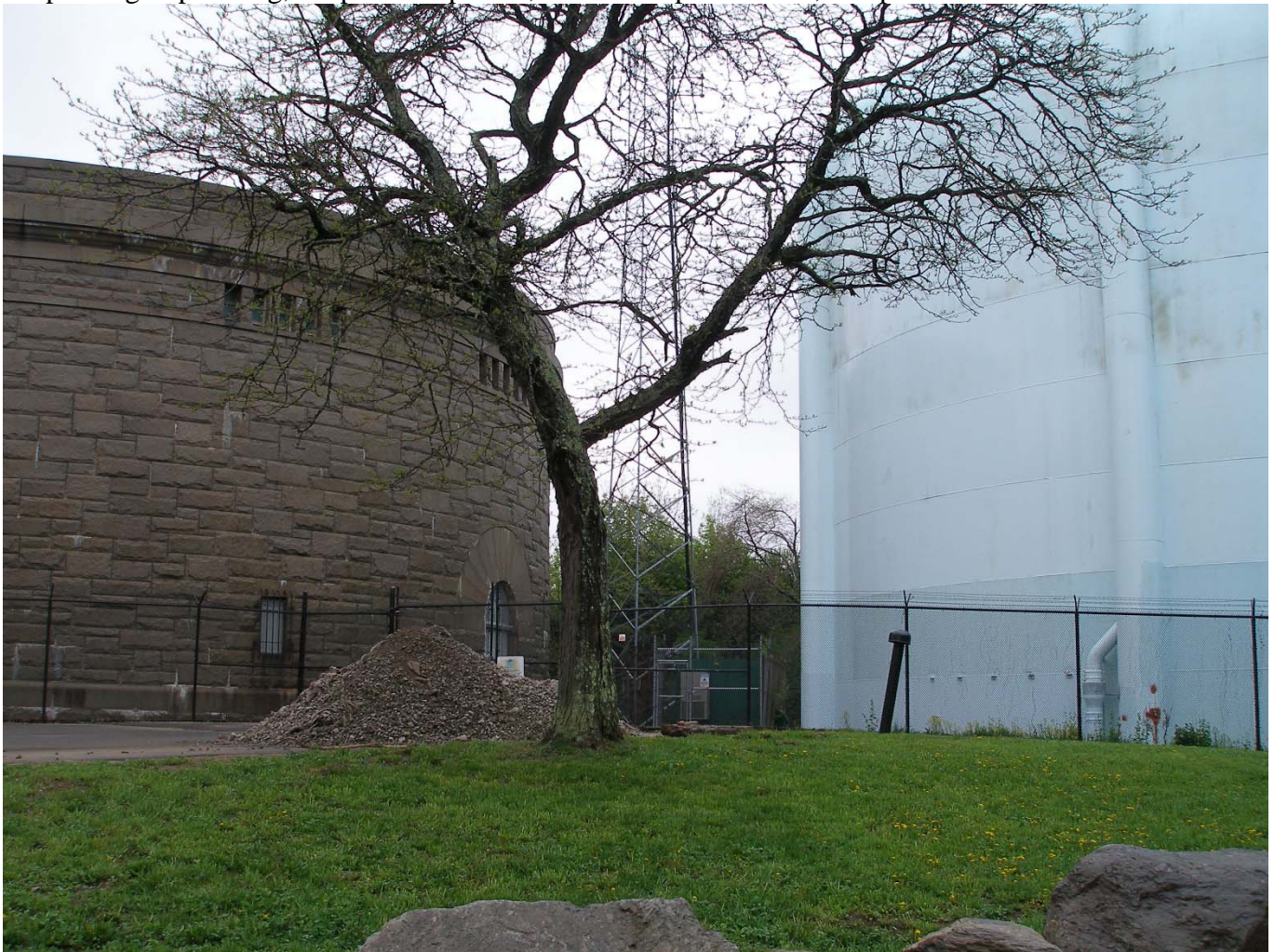
Bellevue Storage Tanks
