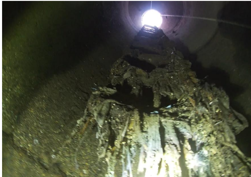
Figure 2-2: Evidence of Surcharge Conditions in the Section 35 SMH
