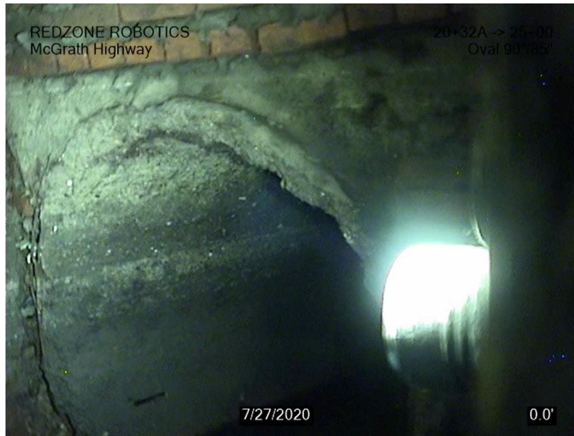
Figure 3-3: CCTV Image of the 42-inch Drain Connection to 85x90-inch Combined Sewer
