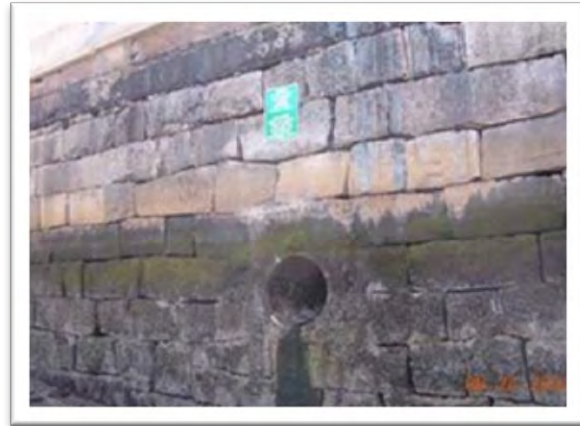
Former CSO Outfall CHE002 now discharges stormwater, only.
