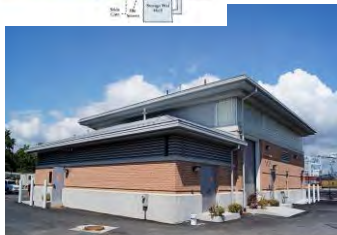
North Dorchester Bay CSO Storage Tunnel Dewatering Pump Station, Conley Terminal, South Boston
