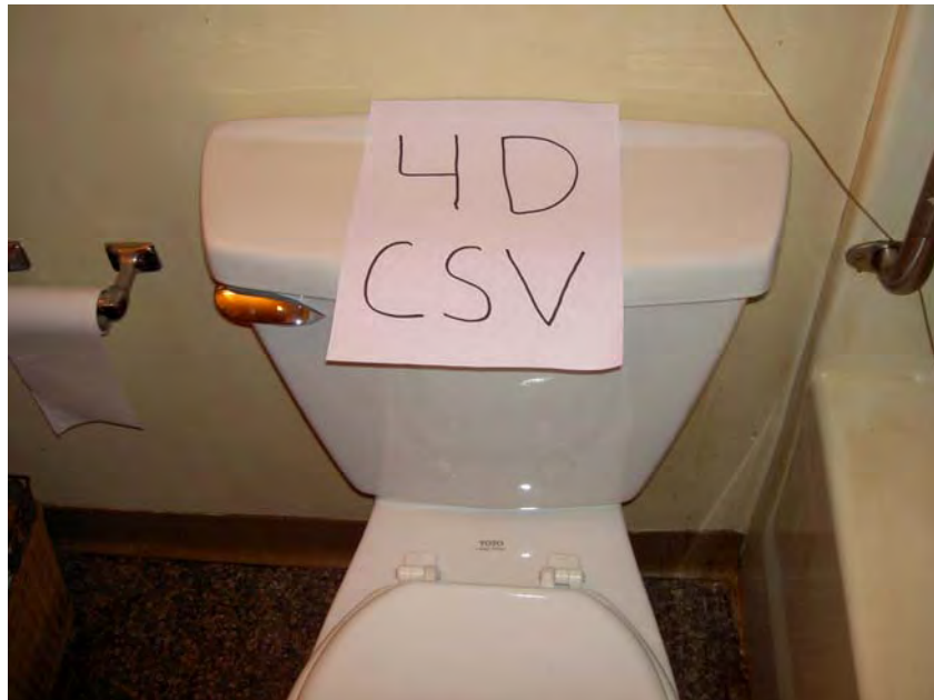
Figure 3.4 Sample Low-Flow Toilet After Retrofit in a Public Housing Unit
