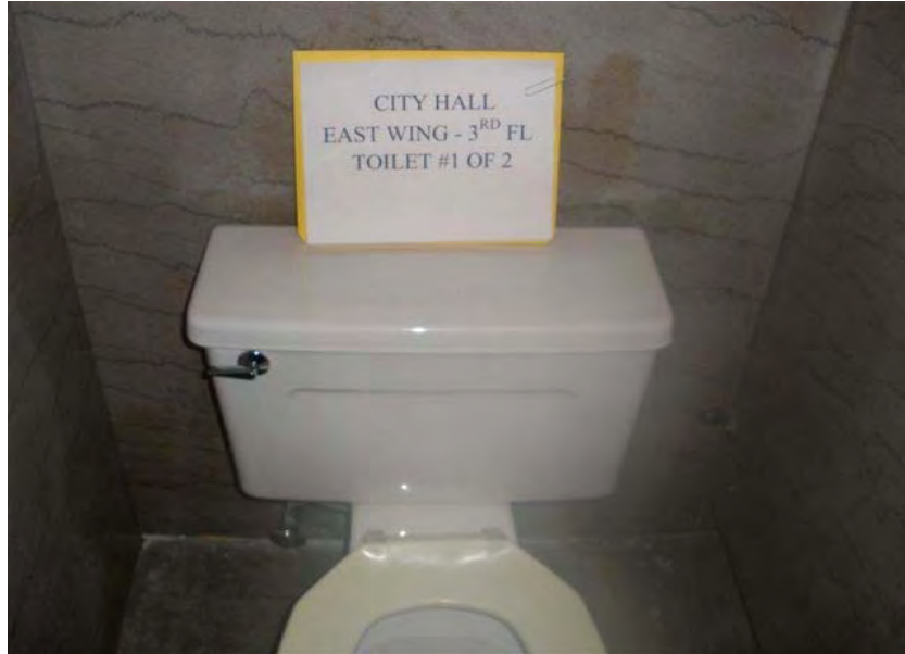
Figure 3.1 Sample High-Flow Toilet Before Retrofit in a Public Building
