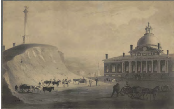
Removing soil from Beacon Hill to provide the proper grade to build the Beacon Hill Reservoir
