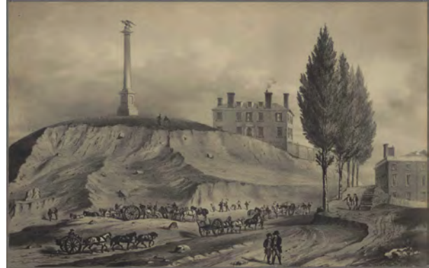
Removing soil from Beacon Hill to provide the proper grade to build the Beacon Hill Reservoir
