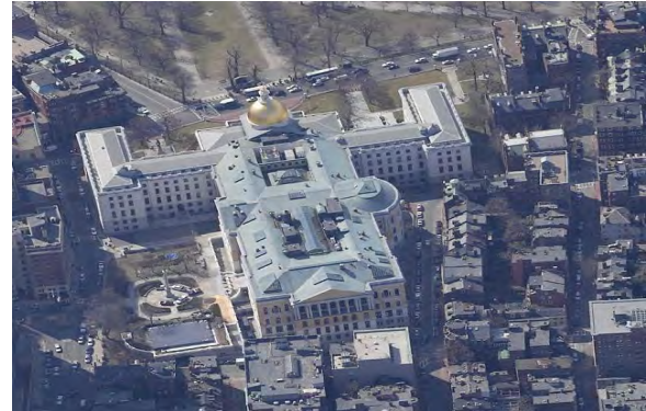
The northern end of the State House Annex extends to Derne St. and is supported by the old reservoir foundation
