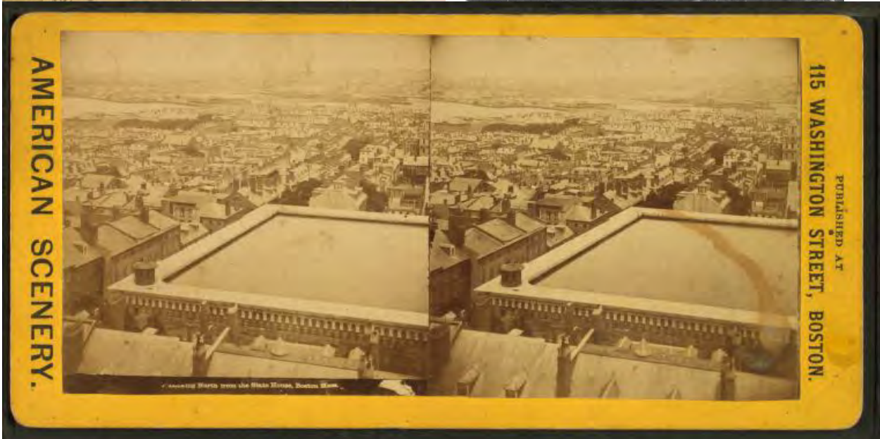
Various views of the Completed Beacon Hill Reservoir
